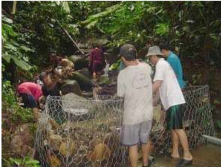
Villagers of Kampung Terian building a dam over a section of the stream for its micro-hydro system project.
