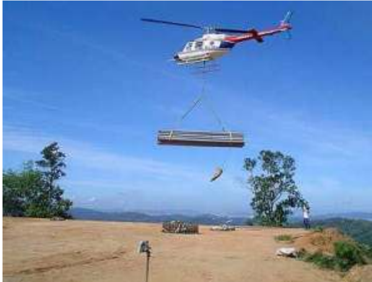
Pipes for the community-based renewable energy project being flown to the interior.
